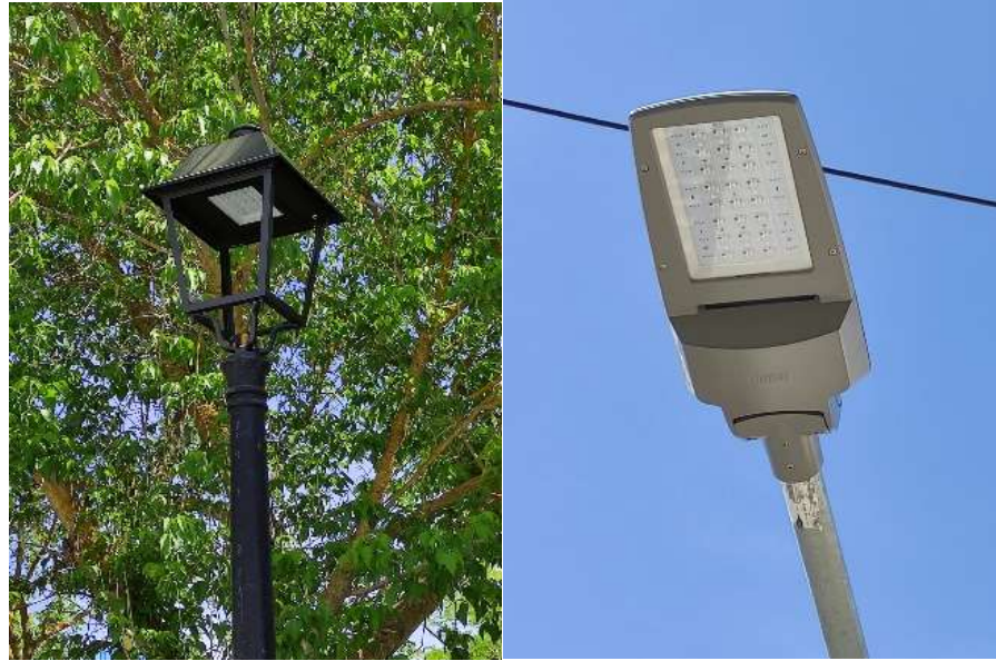
Luminarias led colocadas
